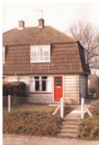
Figure 2 Cornish Unit Type 1 – one of the many types of pre-cast reinforced concrete houses
