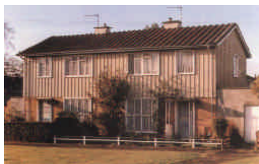
Figure 4 The British Iron and Steel Federation House (BISF)
