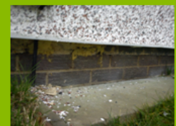
Base rail of external wall insulation system with brick wall between foundations and D.P.C. exposed
