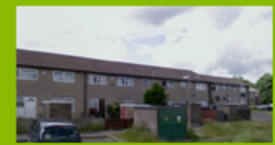
Original Wimpey No Fines Terrace
