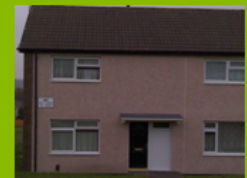
Wimpey No Fines House clad with external wall insulation
